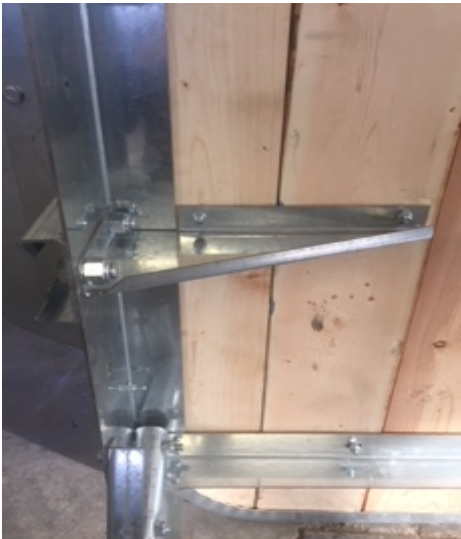
Step 5-Above picture is of the gusset with two 3/8" bolts through the floor and two 3/4" bolts through the skid and frame.
