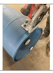
1. Lay the barrel on its side and cut the top off of the barrel approximately 1.5" down from the top. If the barrel top has a ridge in it, you can use that as a guide for the saw guard to rest against. Cut all the way around. If using a Jigsaw, you will need to drill a hole first for the saw blade to go in. Clean plastic shavings off of both pieces with a knife.
